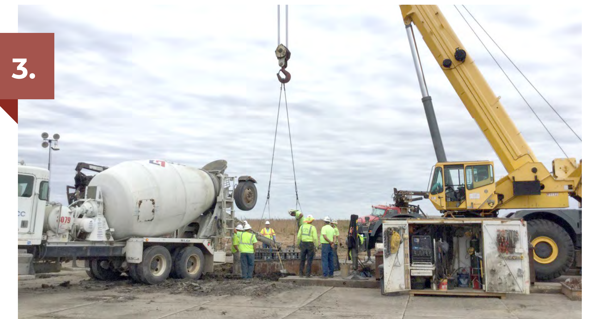
Foundation drilling and pouring
